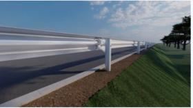
Height-Retaining Anti-Block Device to Upgrade W-beam Guardrails
